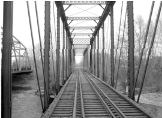
The Rail banked section from 40th ave. out to Naches includes this bridge crossing on the Naches River just east of Glead, next to Highway 12, will be used to create a connection for the Yakima Greenway to our neighbors in Glead and Naches.
