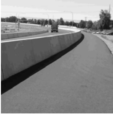
The new bike/ped lane on SR24 Bridge to connect the Greenway on both sides of the Yakima River.
