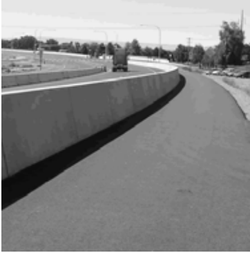
The new bike/ped lane on SR24 Bridge to connect the Greenway on both sides of the Yakima River.
